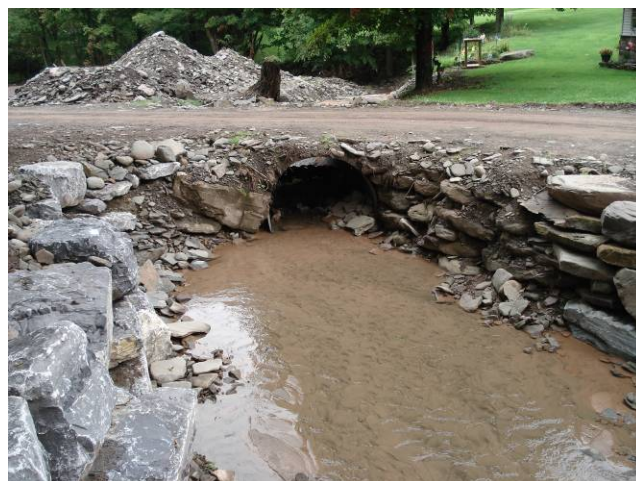
Figure 2.13 Culvert Conveying Holliday Brook
