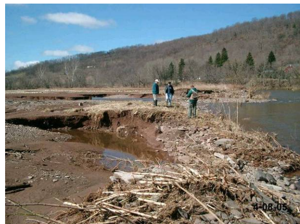
Figure 3.11 Berm that was breached in 2005 storm event
