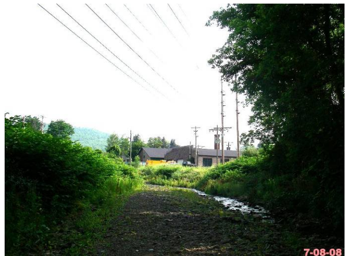
Figure 3.14 Two years later after Post Flood Intervention.
