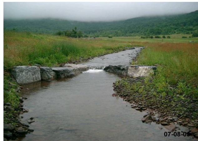
Figure 3.17 Rock Cross-Vane
