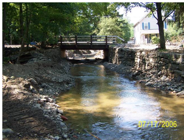
Figure 2.14 Bridge with no floodplain
