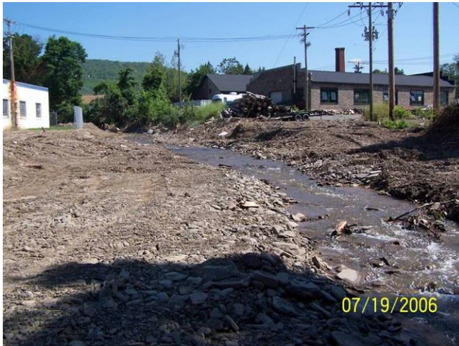
Figure 3.13 Shows stream channel after Post Flood Intervention.
