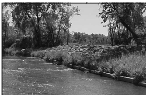
The completed restoration project JB 8-62 on Cazenovia Creek.
