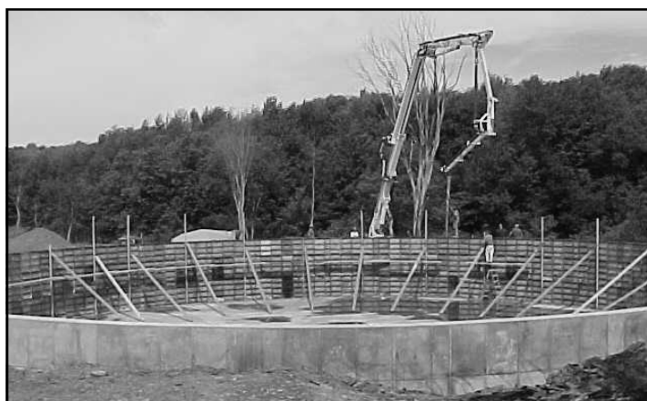
Concrete manure storage lagoon under construction in the Upper Buffalo River Watershed.
