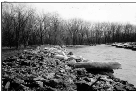
This project site on Cazenovia Creek in West Seneca was designed to minimize damage from ice and was put to the test this past winter. As shown in the photo, it was successful!
