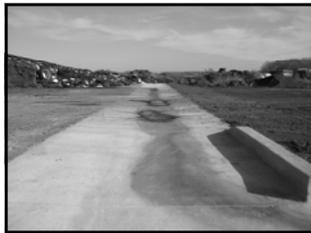
Silo Bunk With Concrete Collection Swale
