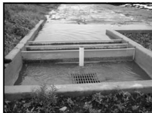
Collection Box to Separate & Transfer Effluent
