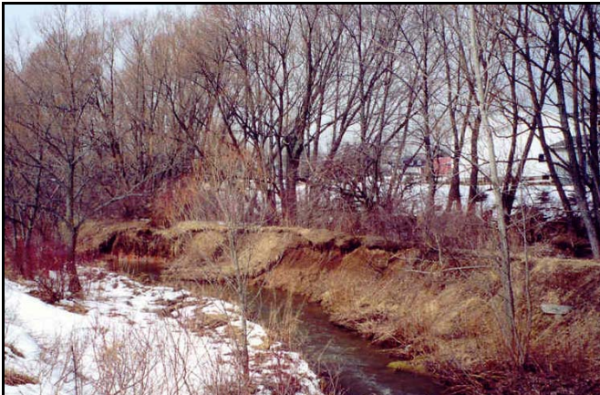
Upstream bank erosion contributes tons of sediment annually to the stream and impairs fish habitat.
