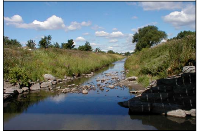
Flood control project between North Creek and South Creek Roads in Cheektowaga.
