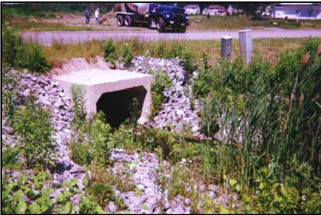
[Map 1 #2] Box culvert at Quail Run development, Lancaster
