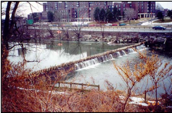
The sill and "finger" dam east of Grant Street, February 2001 (Buffalo State College at rear).
