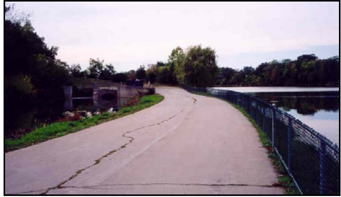
[Map 5 #23] Trash rack (left) and Hoyt Lake (right) in September 2002 after installation of debris-collecting fence
