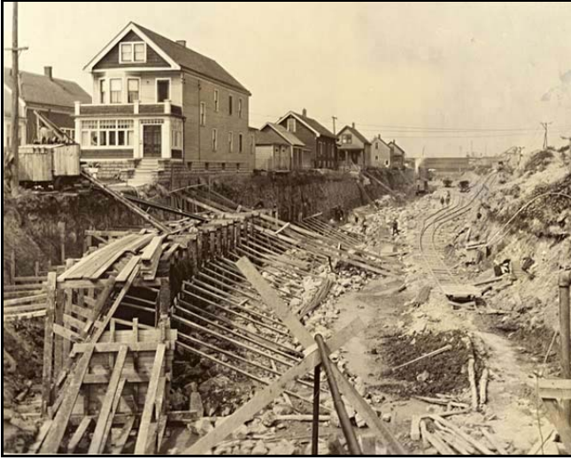
Crews at work on the Scajaquada Drain tunnel project, 1923. (photo courtesy of Western NY Heritage Magazine)
