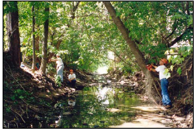
Through a grant from the USDA-NRCS, a tree care crew removed trees in Depew that were threatening property (a home across the stream) and could potentially contribute to soil erosion if the roots were to break free from the streambank.
