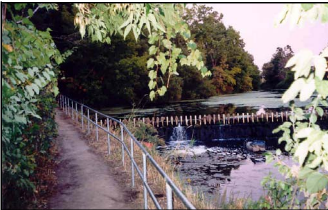
[Map 5 #28] New railing installed in Fall 2002 at finger dam along the Scajaquada Pathway
