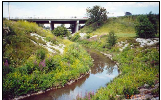
Looking east toward NYS Thruway at Army Corps of Engineers/NYS Department of Environmental Conservation flood control project in Cheektowaga.
