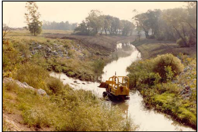
Construction in progress in 1983 on the flood control project near the present-day location of Walden Galleria. (photo courtesy of Edwin Merriman)
