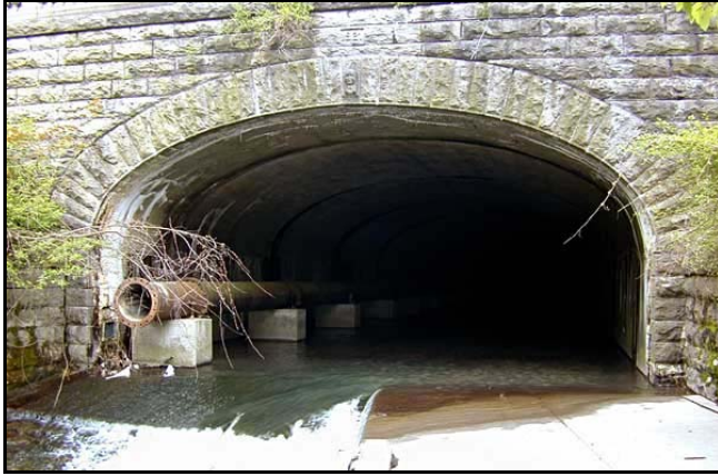
Scajaquada Creek tunnel exit at Forest Lawn. The sewer discharge pipe is at left in the tunnel.
