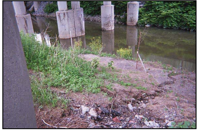
[Map 5 #29] Rill erosion on the streambank along the recreation path under Scajaquada Expressway
